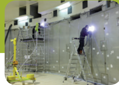
Welding in the water storage pool
