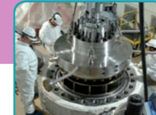
3 High-performance reactor coolant pump for improved efficiency
