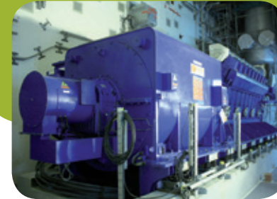
Emergency diesel generators
