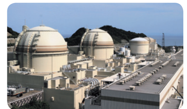
Ohi nuclear power plant, Japan Photo courtesy of Kansai Electric Power Co., Inc.
