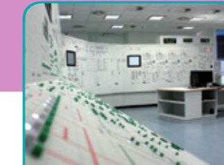
4 Control room with advanced digital I&C systems
