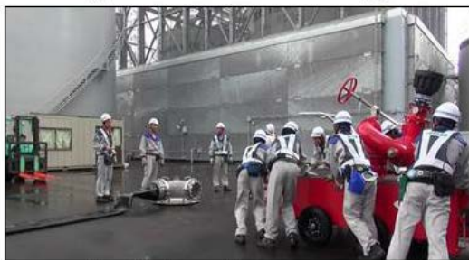
Installation of water cannon
