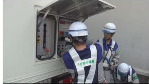
Power cable connecting to the high voltage generator
