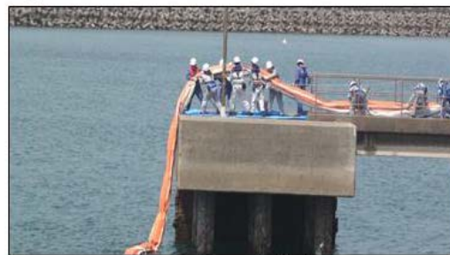
Installation of silt fence
