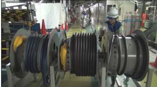
Power cable laying (inside the building)
