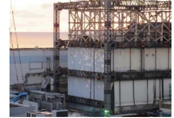
Panels removal completed (Nov. 2016)
