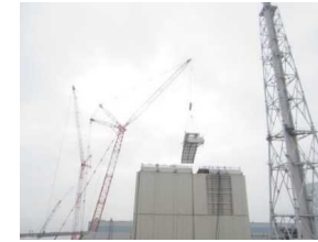
Removal of roof panels (Jul. 2015)
