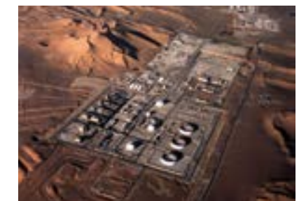
Natural Gas Facility
