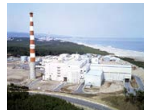
Nuclear Fuel Reprocessing Plant for JAEA
