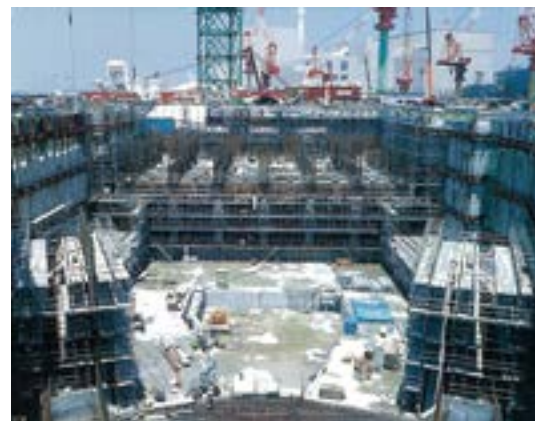
Intake Pond Structure (Design & Construction)
