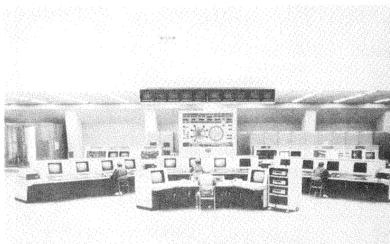
Central Control System of "JT-60"
