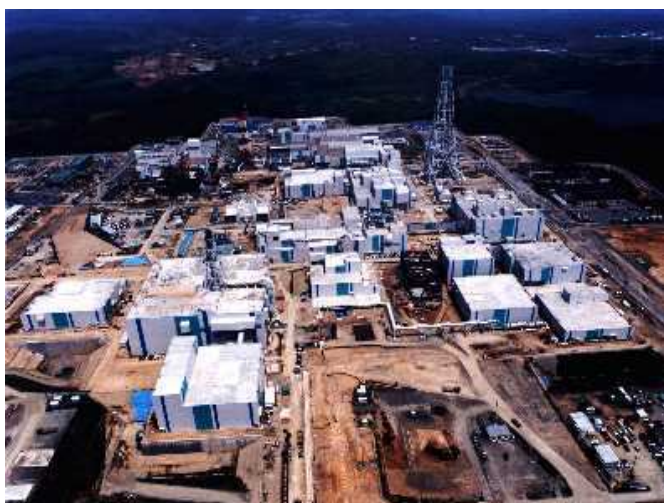
JNFL's Rokkasho Facilities
