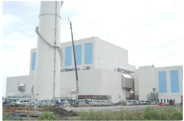
Tohoku Electric Power's Higashidori-1 NPS
