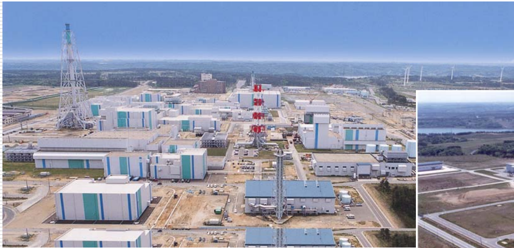
Rokkasho Reprocessing Facility
