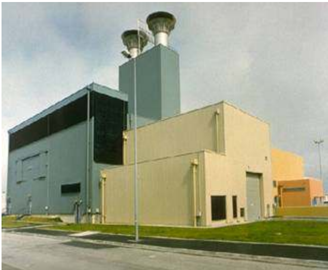
Temporary storage, La Hague
