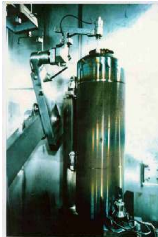
Canister of vitrified products
