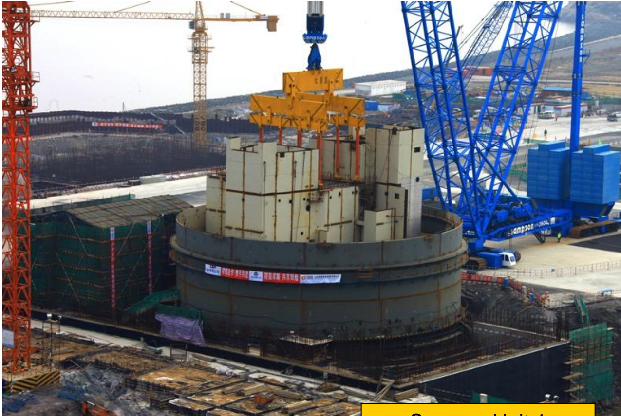
Sanmen Unit 1 March 27, 2010
