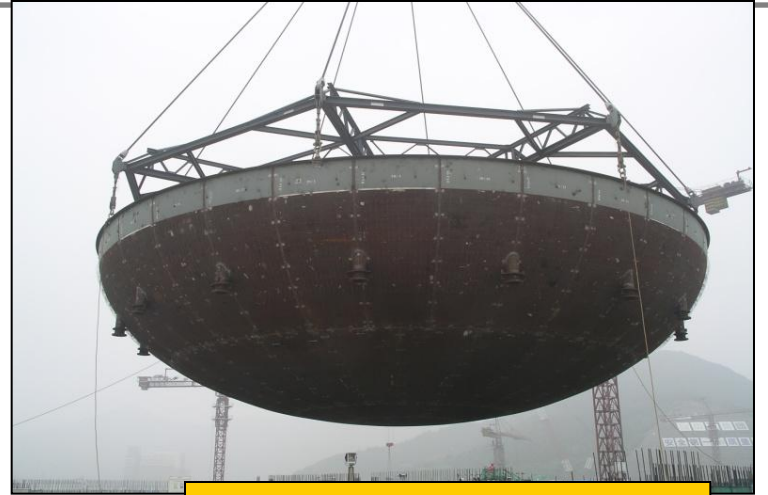
Sanmen Unit 2 June 13, 2010
