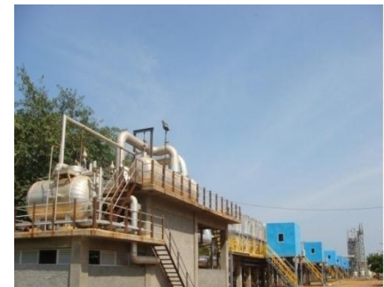
NUCLEAR DESALINATION DEMONSTRATION PROJECT, KALPAKKAM, TAMIL NADU
