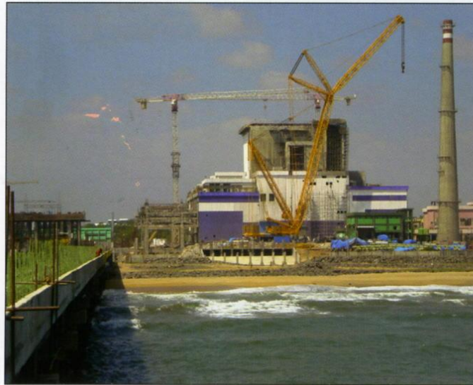
Fig. 1 Overall view of nuclear building
