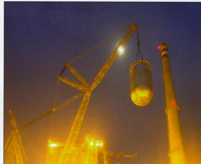
Fig. 2 Erection of main vessel of PFBR
