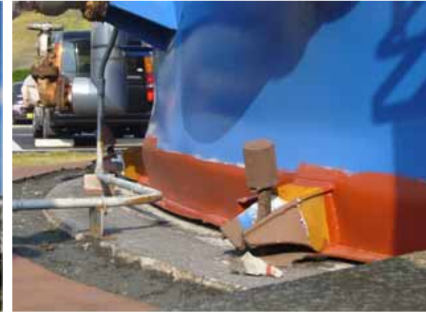
Filtration Tank Seismic class: C Status : Buckling
