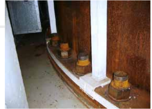
Sound anchor bolts for RPV (As)
