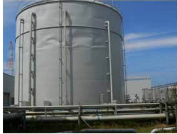
Deionized Water Tank Seismic class: C Status : Buckling
