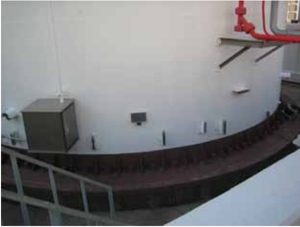
Petrol Tank Seismic class: As “equivalent” Status : No damage
