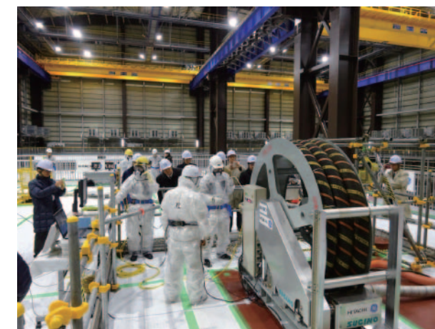
Photo 1: Implementation of reinforcing workability verification test for S/C support columns
