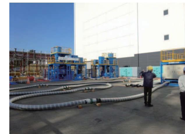
Photo 2: Supply equipment of reinforcing material for S/C support columns (outdoor)
