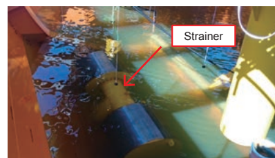
Strainer before injection of concrete
