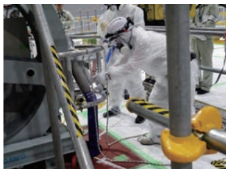
Lowering hose operation into a mock-up torus room
