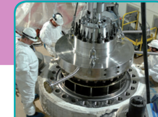
3 High-performance reactor coolant pump for improved efficiency
