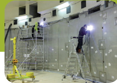
Welding in the water storage pool
