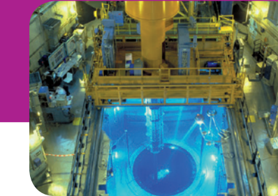
Reactor fuel loading
