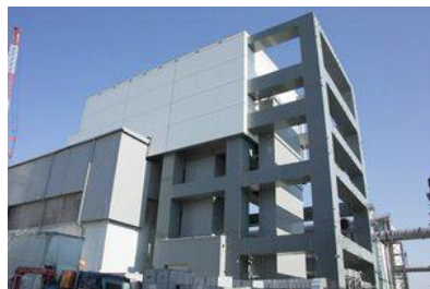
Equipment for fuel removal
