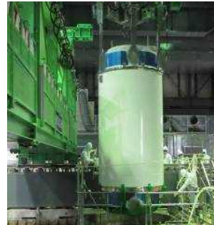
Storage of removed fuel
