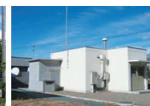
Takasaki monitoring station (measurement of particulates and noble gases)
