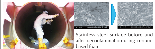
Figure 1. Chemical Decontamination for Vacuum Truck in Fukushima Daiichi NPP
