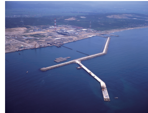
Kashiwazaki-Kariwa Nuclear Power Plant
