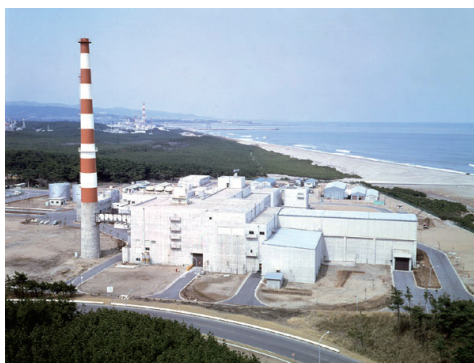
Nuclear Fuel Reprocessing Plant for JAEA
