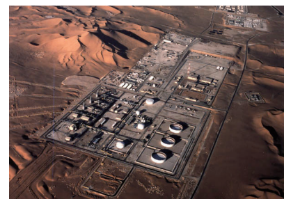
Natural Gas Facility
