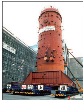
Transportation of Pressurized Fluidized Bed Boiler (3,820 tons) for a Thermal Power Plant
