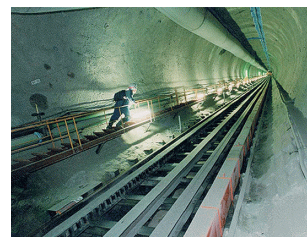
Kannagawa Hydropower Station
