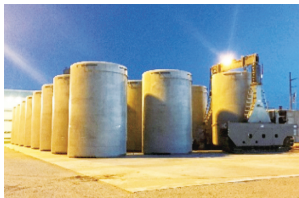
Dry Storage Systems (Concrete Cask)
