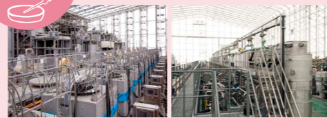
Multi-nuclide removal equipment (ALPS)
