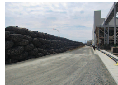
Existing seawall (2.4-4.2 m)
