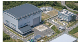
Naraha Center for Remote Technology Development (Naraha Town)
