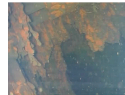
Inside primary containment vessel
