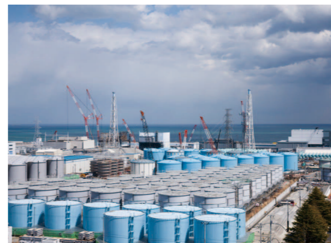
Approx. 900 tanks have been installed in a planned fashion (Each tank stores approx. 1000-3000 tons)
