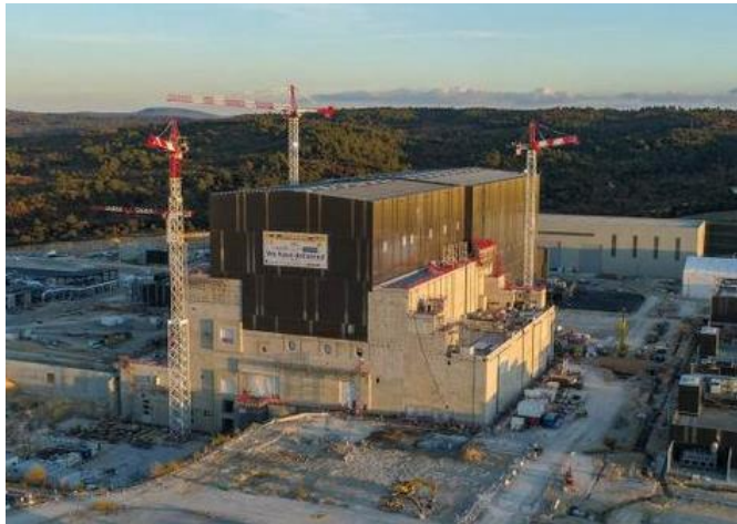
Tokamak Construction (Nov 2020)
