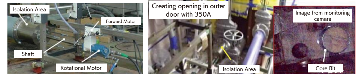
▲ Creating opening in outer door of airlock with core opening equipment (Figure 3-2)
