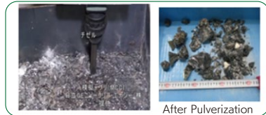
▲ Pulverizing debris with a chisel; mixture with water due to crevice expansion
