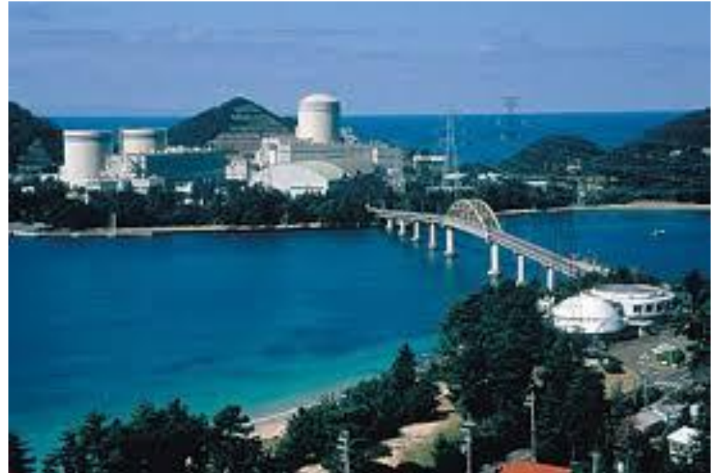
Mihama Nuclear Power Station Source: Kansai EPCO
