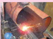
Utilization of thermal cutting (gas cutting) [Turbine system piping cutting]
