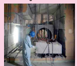
Utilization of mechanical cutting (wire saw) [Through-holing work to the building]
