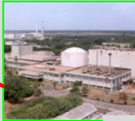
FBTR, 40 MWt, 13.5 MWe, Loop type (Pu-U) Cfuel, in operation since 1985
