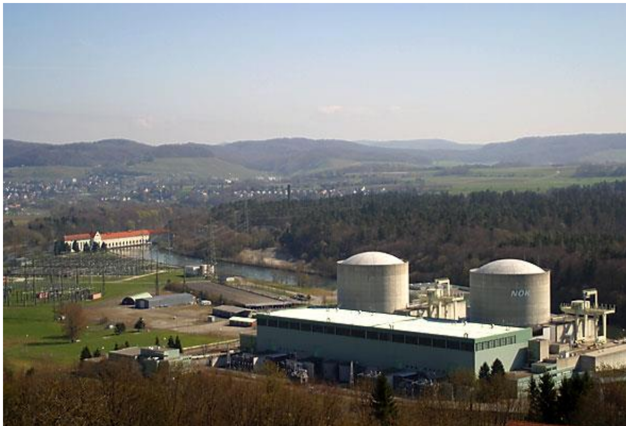
Beznau nuclear power plant
