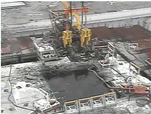
Removal of Fuel Handling Machine from SFP (Aug. 2015)
