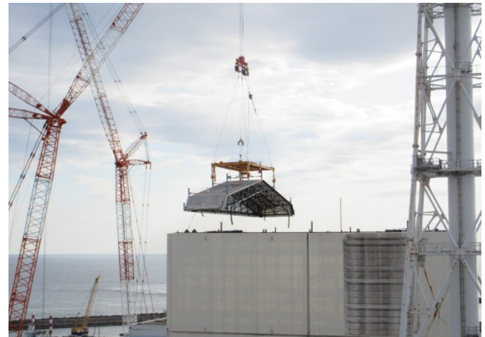
Reactor building cover
