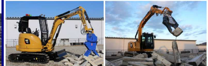
Small and large wireless heavy machine (removal of debris indoors and outdoors)
