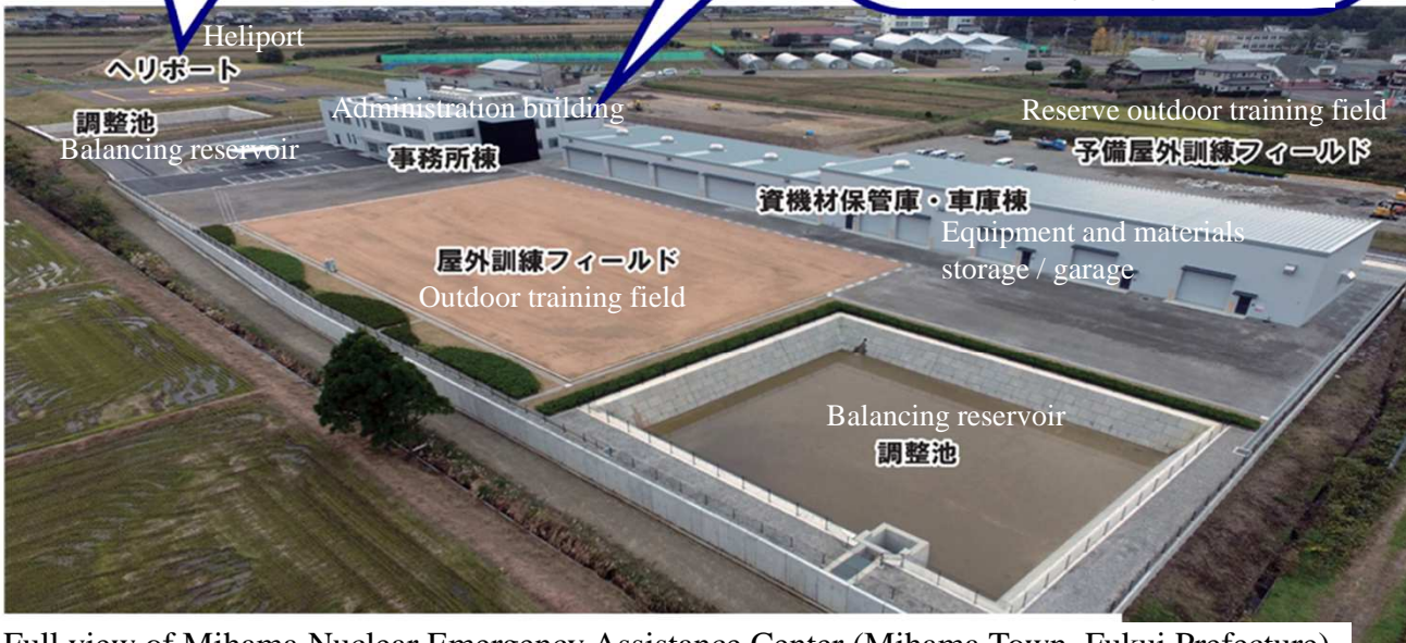
Full view of Mihama Nuclear Emergency Assistance Center (Mihama Town, Fukui Prefecture)
