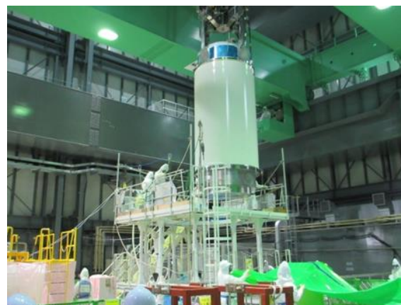
Process of removing fuel rods at SFP Unit 4
