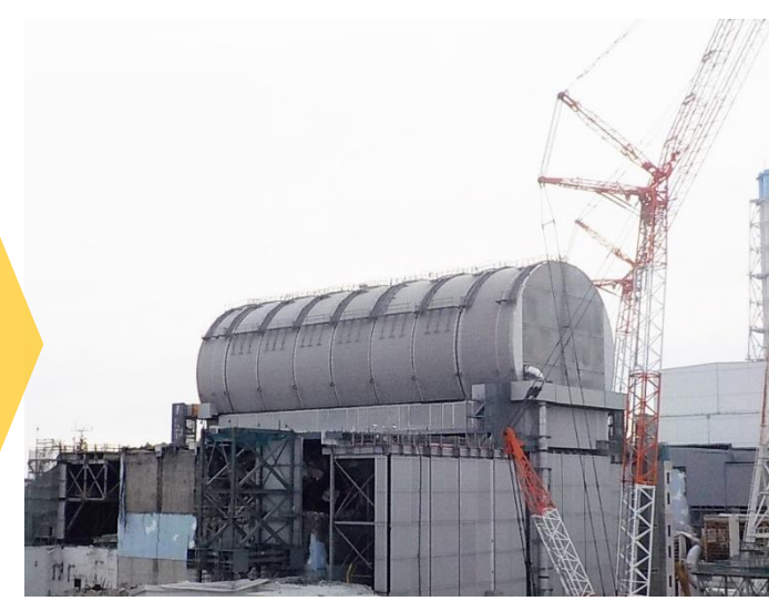
Installation of a dome roof
