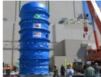
Filtered venting system (Reference: HP of Chubu Electric Power Co.) R/B hydrogen ventilator
