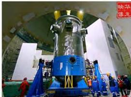
The reactor pressure vessel has been installed at China's demonstration Hualong One nuclear reactor, Fuqing 5, under construction at in Fujian province.
