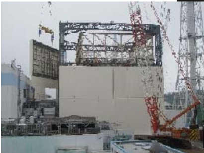
Installation of Reactor Building Cover
