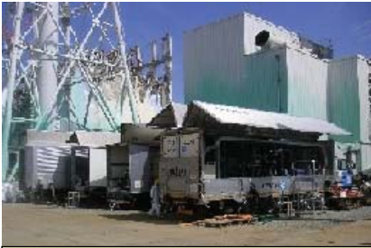
Desalination plant for Spent Fuel Pool Water
