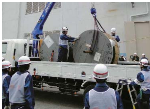
Emergency Installation of the Electric Cables
