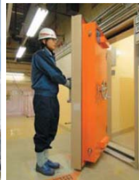
Water tight Doors
