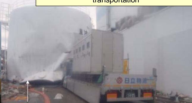
Heavy oil tank washed away by the tsunami and blocking the road
