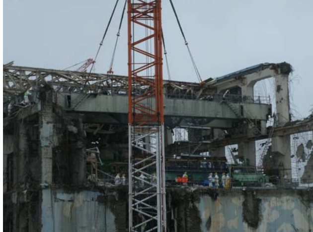
Removing rubble from Unit 4
