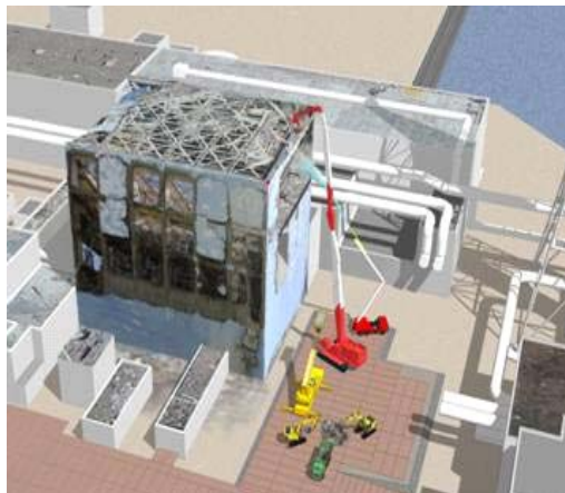
Removal of Rubble
