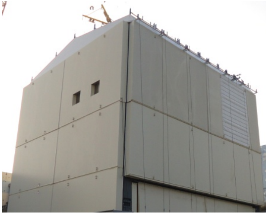
Installation of the reactor building cover on Unit 1
