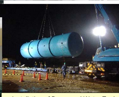
Installation of Processed Water Tank
