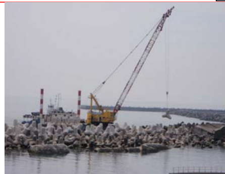
Restoration of Breakwater
