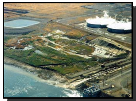
Waterborne release at Hanford Site, Washington State, 1963
